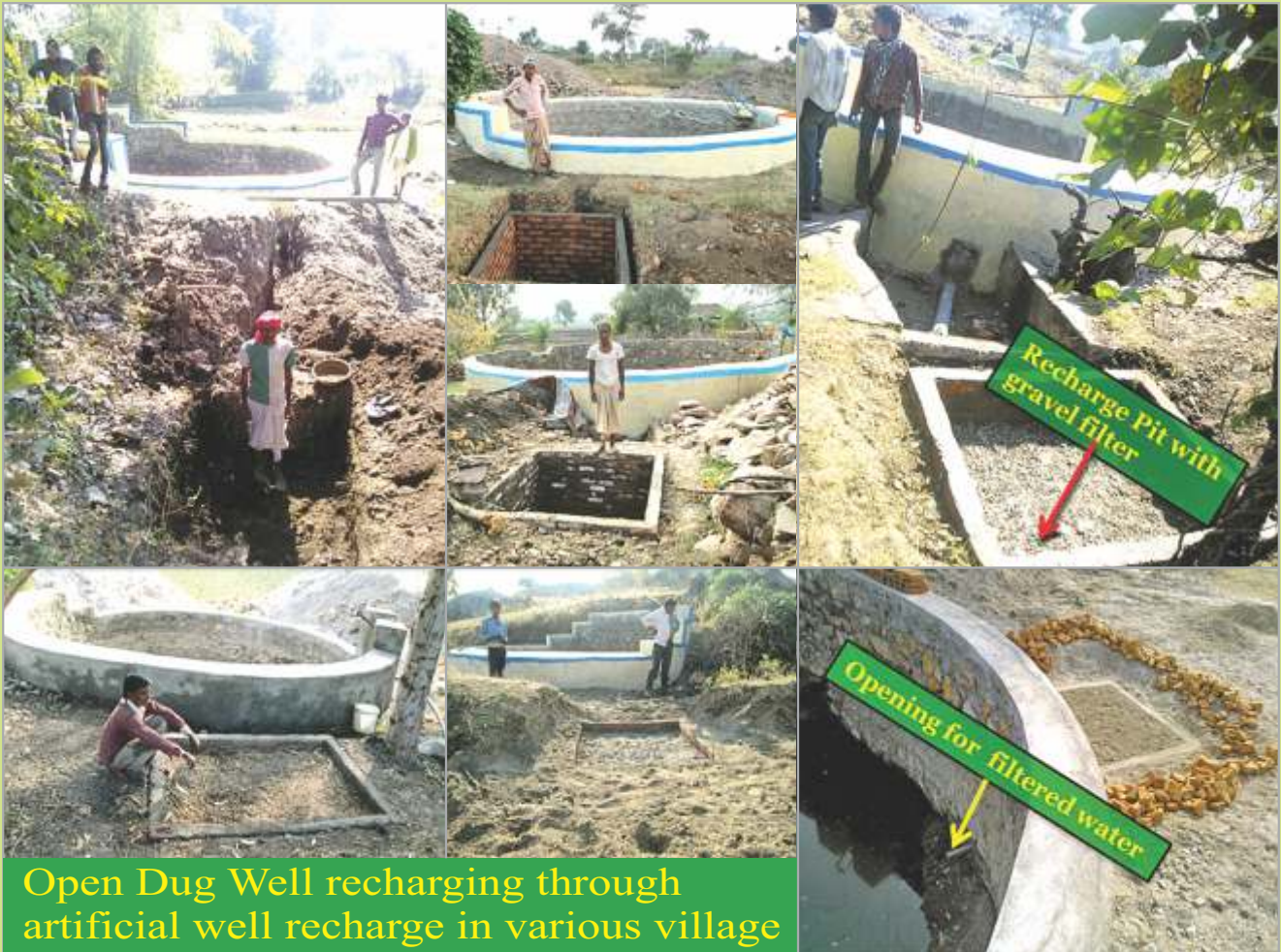
Artificial recharging of wells under Watershed Development Programme in district Banswara, Rajasthan under Coca-Cola India Foundation
